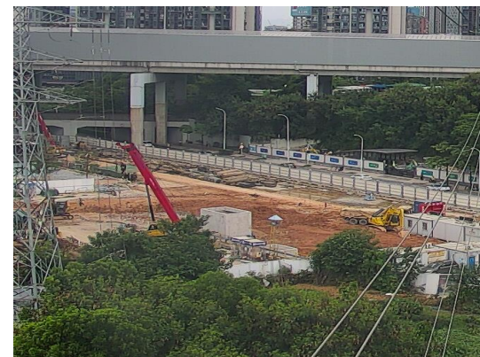
吊车：无效告警
